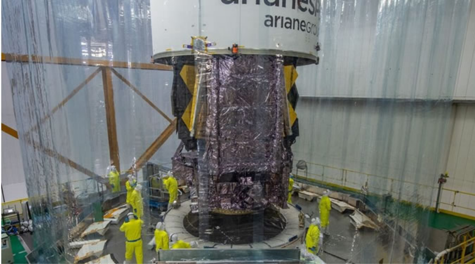
NASA's James Webb Space Telescope being encapsulated within the Ariane 5 payload. Credit: ESA/CNES/Arianespace
